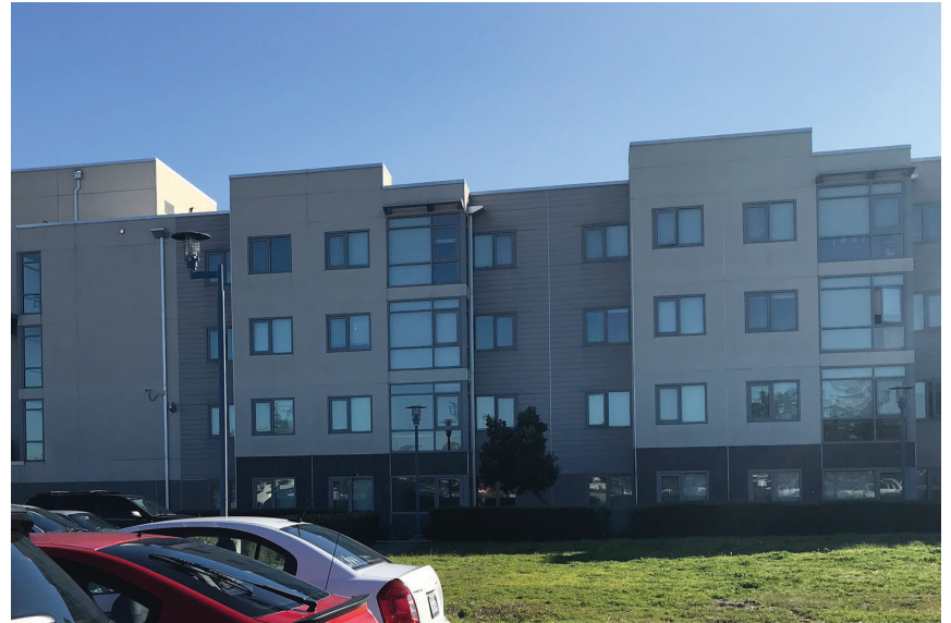
North Quad Housing (Main Campus)
